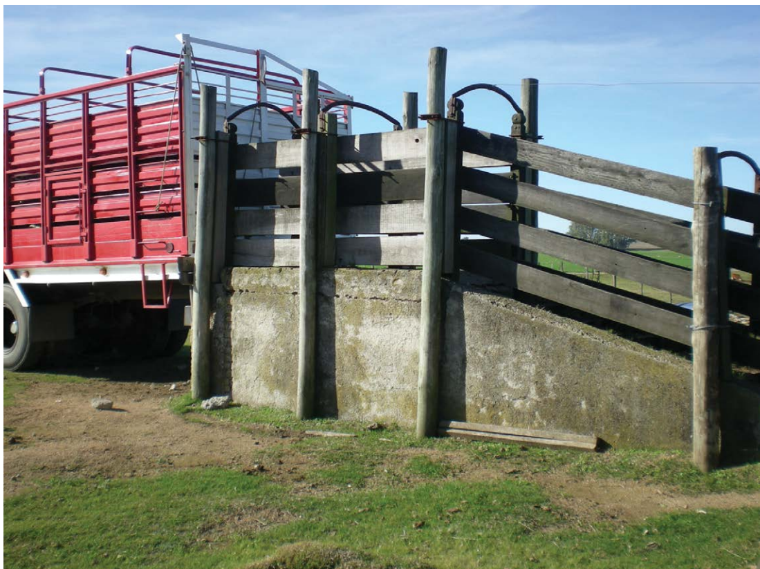
Fig. 19.1. Some of the worst welfare problems associated with transport occur during loading and unloading. Good facilities for these procedures allow animals to enter or leave the transport on the level, or by a gently sloping ramp with good footing, and with races and barriers that encourage quiet movement. Such facilities need not be expensive to construct.
